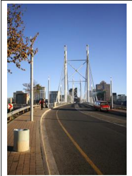
Nelson Mandela Bridge, Johannesburg, sent by Nikkie
