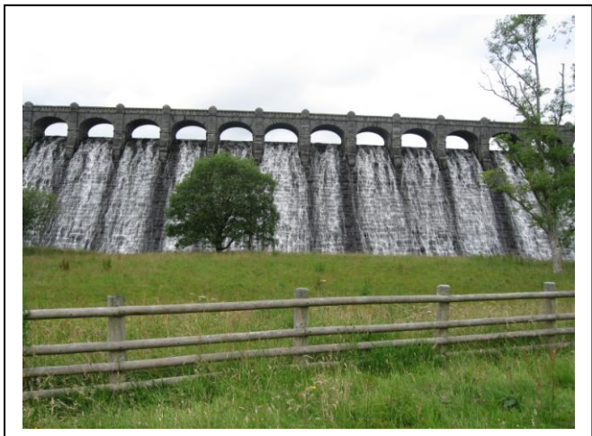
Bridge in Wales sent by Marlies Witthagen, AC The Netherlands
