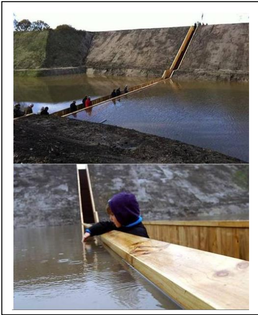
The Moses Bridge, The Netherlands
